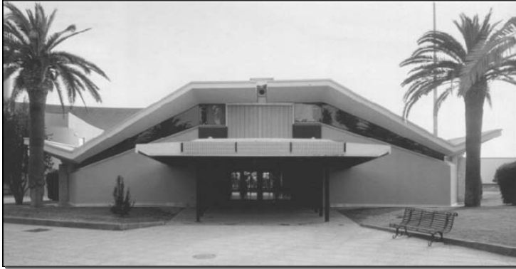
Figure 2 - The building after the addition of the cladding walls.
