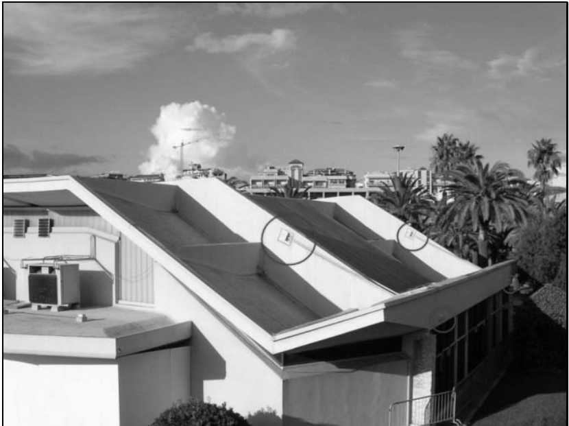
Figure 29 - Ties in the upper part of the beams.
