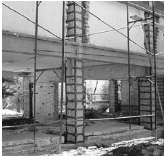
Fig. 1 - R/C columns strengthened by means of angles and battens.
